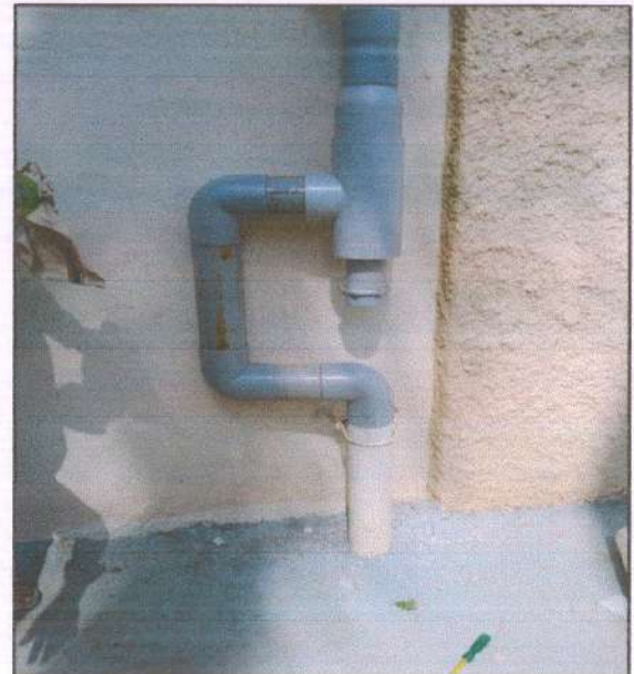
One line filter system provided for Rain Water Harvesting.
