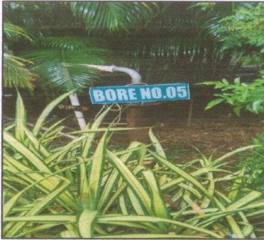
Piezometer installed at Borewell No. 5
