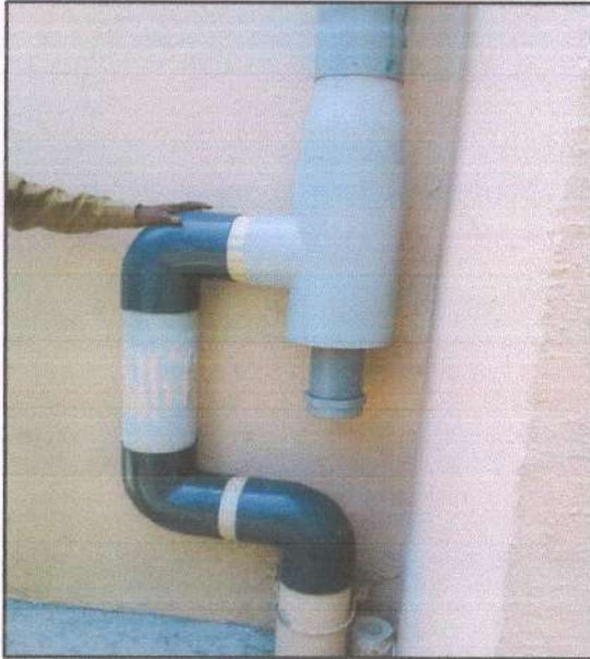
One line filter system provided for Rain Water Harvesting.
