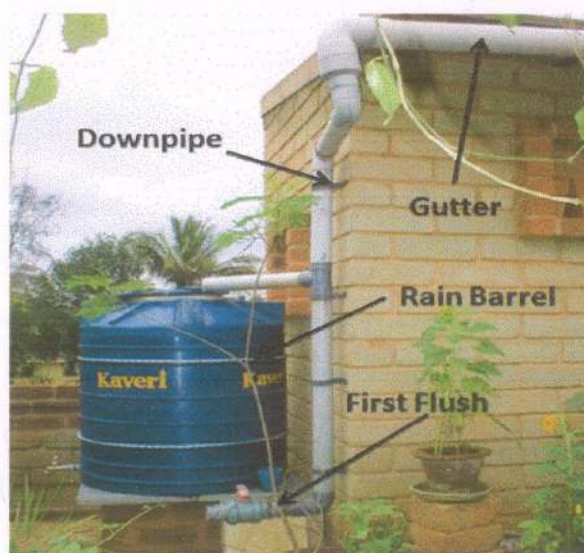
Fig. 3.1 Storing rain water for direct use
